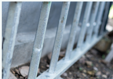
Check rungs and rail condition
